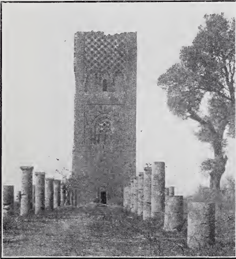
The largest mosque ever attempted by the Moors was located in Rabat. This picture shows about all that remains of the building. This tower had a roadway instead of stairs so that the muezzin could ride a donkey to the top when he went to call the faithful to prayer. The ruin is known as Hassan Tower.
